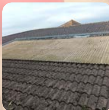
Roof - before and after!
