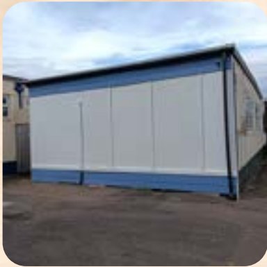
The exterior side of the iZone has been cladded
