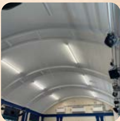
The ceiling in the Drama Hall has been patched and painted
